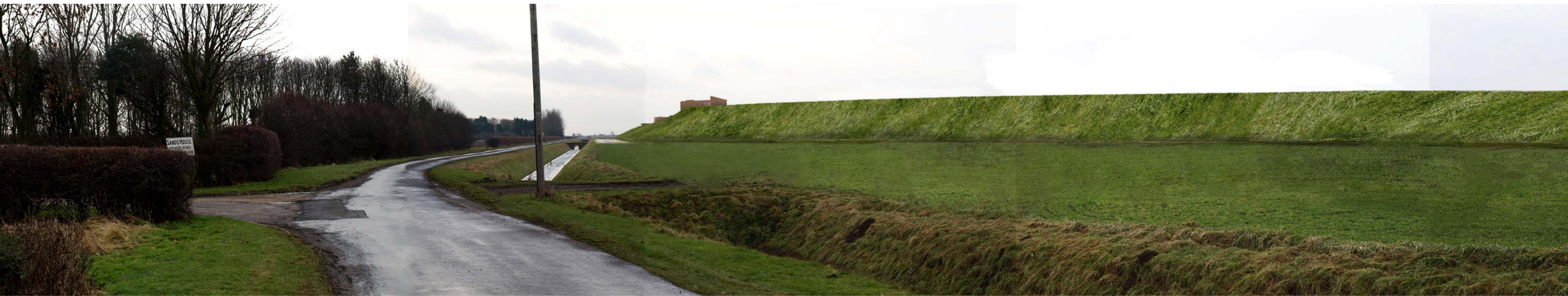
Photomontage No.1: View taken from Cherry Cobb Sands Road approximately 4 metres from the site looking south east
